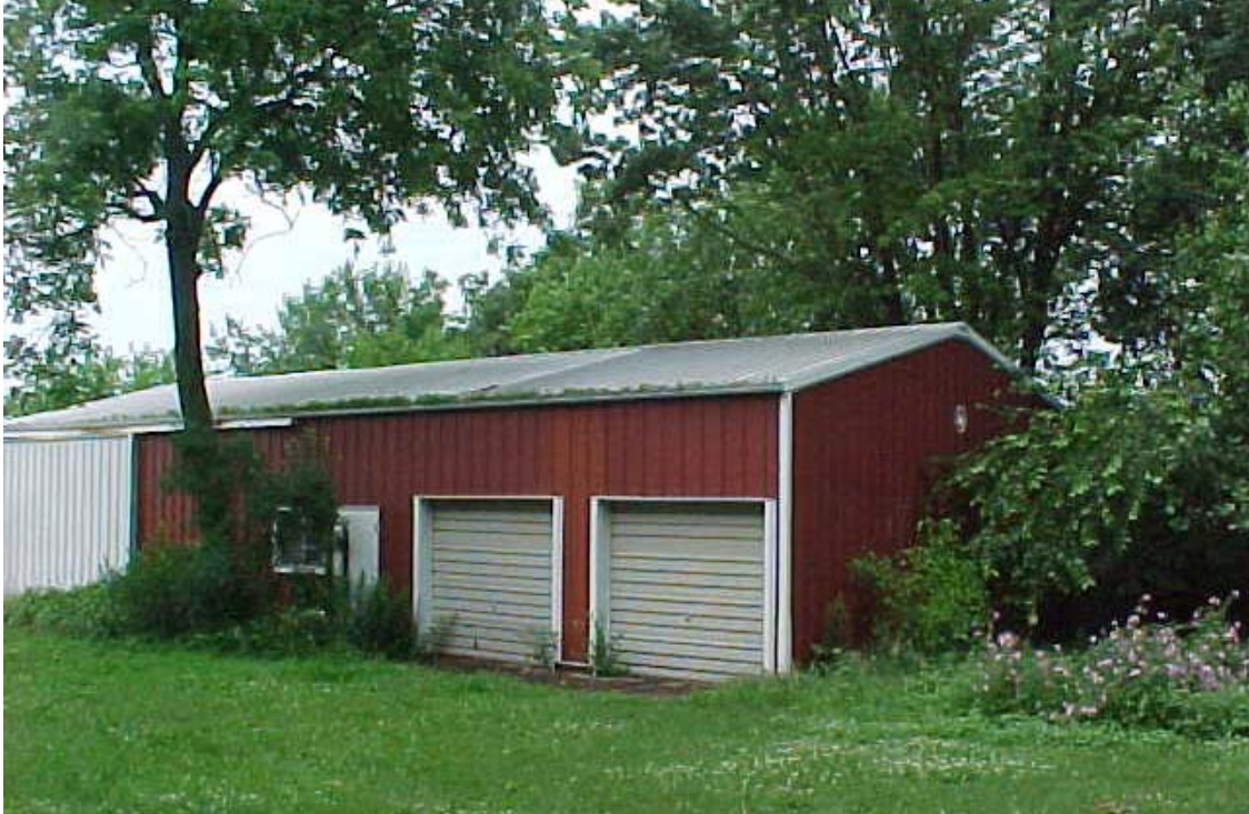
West Machine Shed
